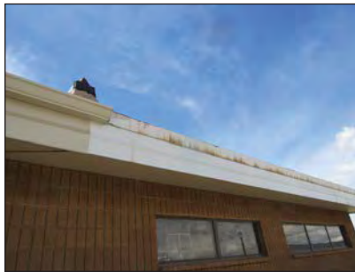
Replace missing gutters
