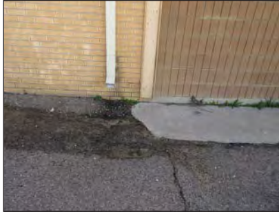
Replace missing downspouts
