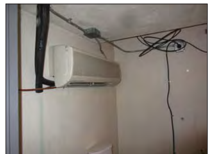
All wiring needs to be cleaned up
