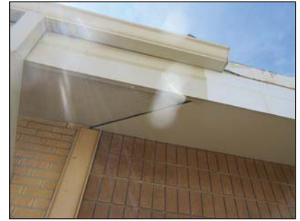
Repair/replace metal flashing
