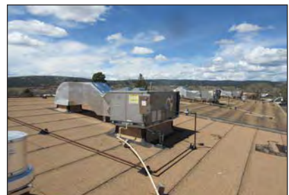
Reroute condensate lines
