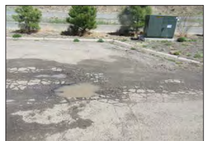
Pavement deteriorated
