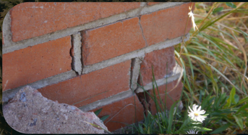
Cracks go all the way through building
