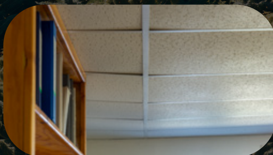
Ceiling has warped and is sinking
