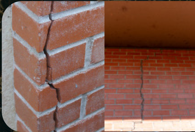
Cracks go all the way through building
